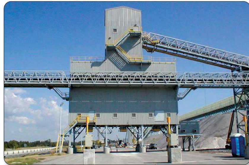
Triple bay truck loadout system
