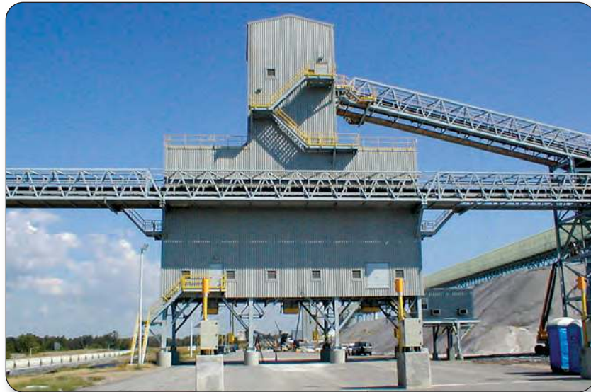
Triple bay truck loadout system
