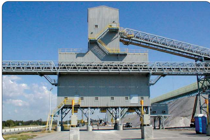
Triple bay truck loadout system
