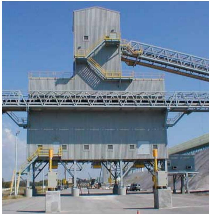
Figure 5. Automated multiple bay truck loadout.
